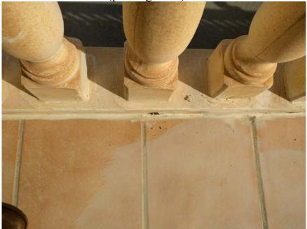
We have also observed that in different lateral courtyards of certain dwellings no maintenance has been performed, and therefore, at first sight, there is a lack of joint treatment between the different pieces, which also contributes to the different leakages detailed in the photographic documents attached herein.
