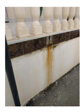
We may observe quite clearly the cracking of the joint seals and therefore water leakage through them, due to the absence of a waterproof membrane that must be vertically extended in the joint of the façade of the dwelling and the exterior paving.
