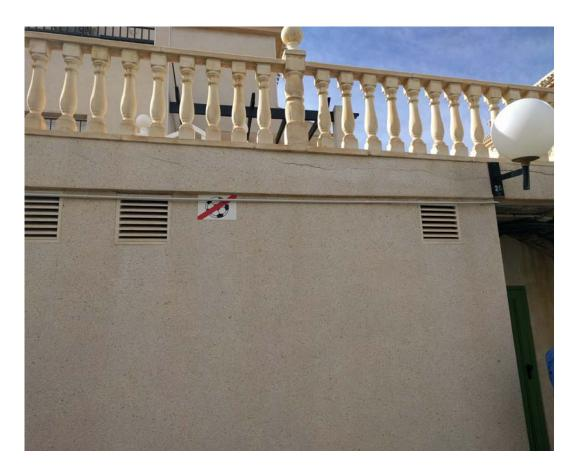
We have observed that the exterior air intakes are at the same height as that of the asphalt irrigation, which causes the entry of water directly, leading to the existing dampness.
