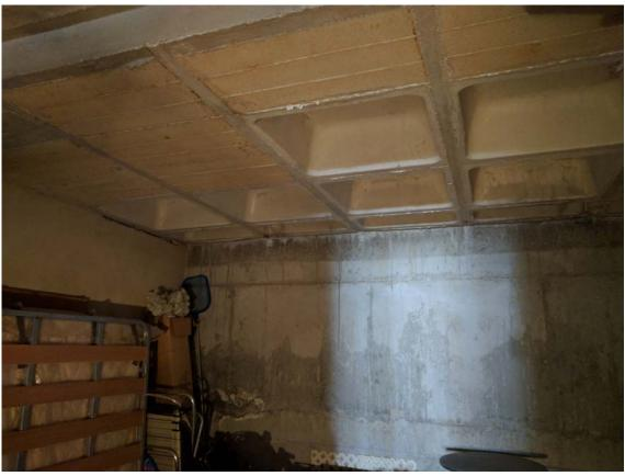
In the inspection performed, we have been able to check the poor state of the expansion joint that, although it was once repaired and masked with a metal "crackfiller", a new adaptation should be considered, due to its bad execution.
