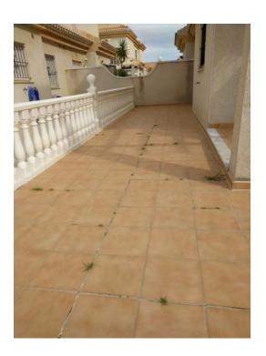
In different points of the floorings of corridors between dwellings, we may observe, at first sight, certain areas in which, due to their overpass, water accumulates without subsequent draining and, therefore, it contributes, as we said before, to the leakage of water to the parking units.
