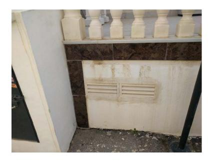
On the superior left angle we may see the poor finishing of the joints of the faces as well as the loosening to which we referred to as in the previous photographs.
