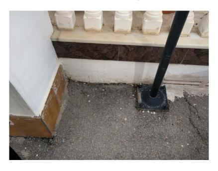
Following with the usual keynote within the joint seals of the façades of the dwellings, we see the loosening of the finishing mortar near the area where the parking area has been built.
