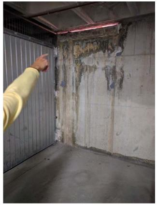
**Interior vertical faces.-** They have not got any kind of finishing, as they are in their primary state, being affected by the dampness from outside, especially in the stairs located on the left said of the parking area by its main entrance, and therefore, it is convenient to repair the damages observed both outside and inside.
